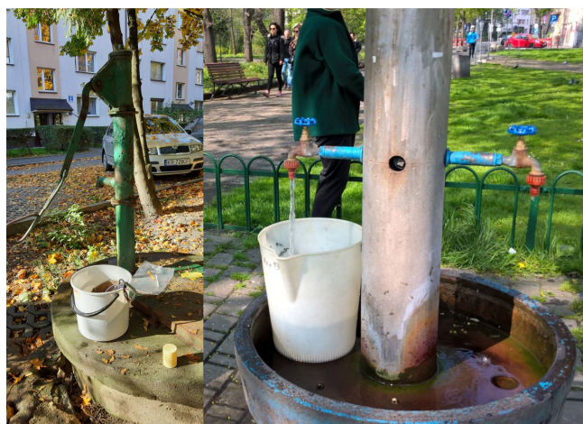
Figure 2. Photographs of representative surveyed wells: left – bored/dug well with piston pump; right – artesian deep well with tap.
