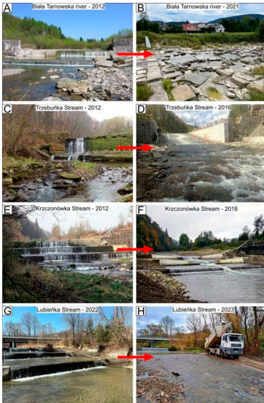
Figure 7. Concrete weir on the Biała Tarnowska river (A) rebuilt into a “honeycomb” type riffle (B); reconstruction of a high check dam on Trzebuńka Stream (C) into a long-roughened riffle serving also as a fish pass (D); and filling of old weirs on the Krzczonówka (E,F) and Lubieńka (G,H) streams with a gravel.
