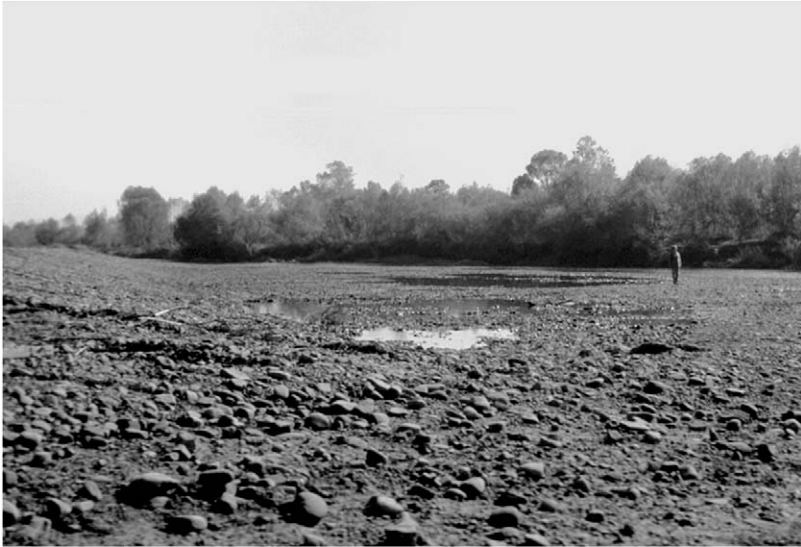
Figure 20.4. Skimming of the gravel bar positioned against an undercut concave bank in the channel of the middle Raba River undertaken in order to eliminate flow confinement and move the thalweg away from the bank.
